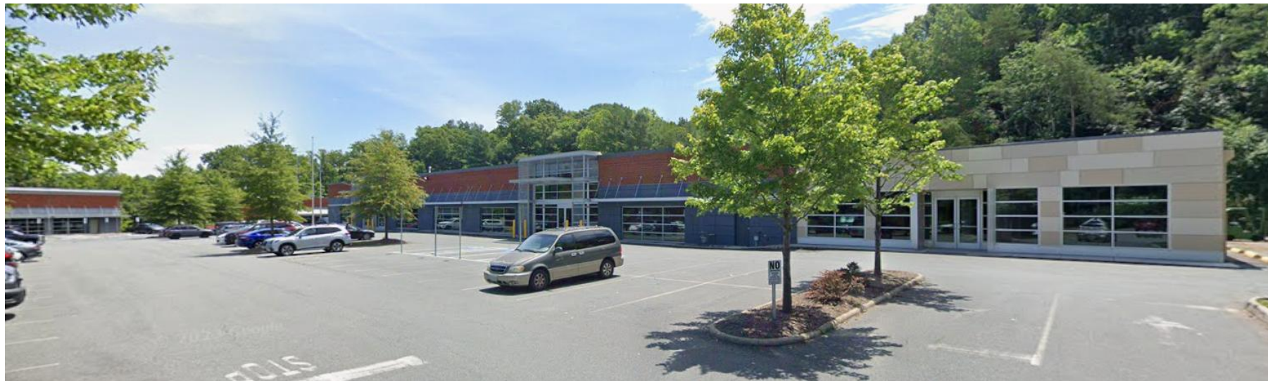
Figures 3a & b: Google street views of Building #2325 prior to renovation for medical offices (top) and after (bottom).
