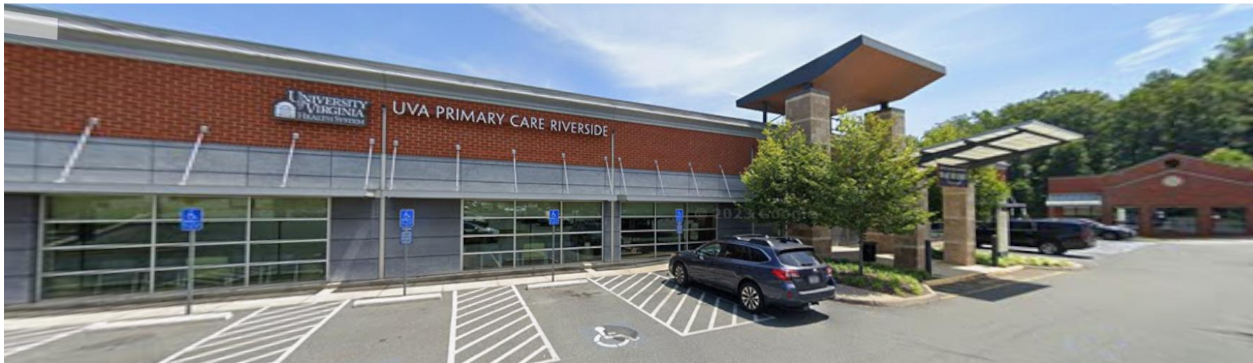
Figures 2a & b: Google street views of Building #2335 prior to renovation for medical offices (top) and after (bottom).
